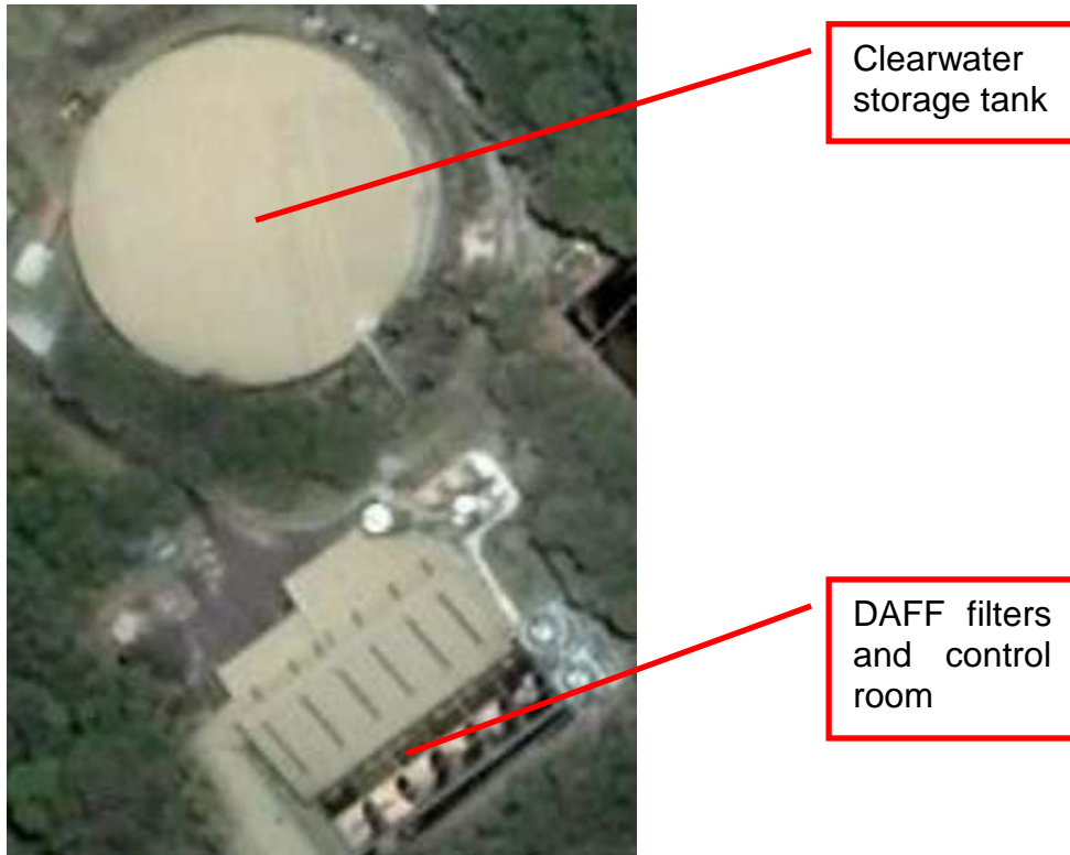
Figure 11: Satellite image of Nightcap WTP
