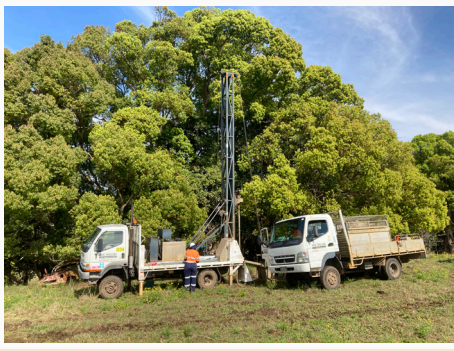
Geotech investigation shows some areas are still unstable.
