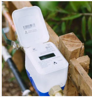
A new smart meter is installed.
