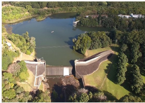
Emigrant Creek Dam.
