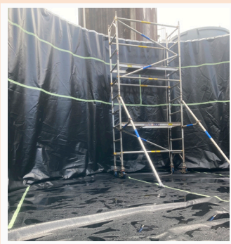
Liners were installed in three critical tanks.
