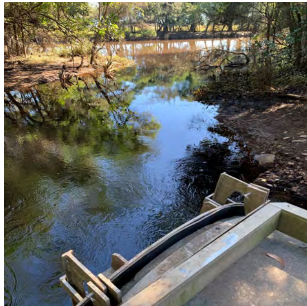
Blackwater discharging from a drainage system at Bungawalbyn in April 2021
