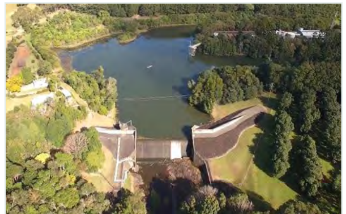
Emigrant Creek Dam
