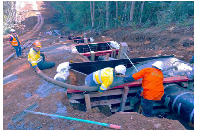
St Helena water pipeline works
