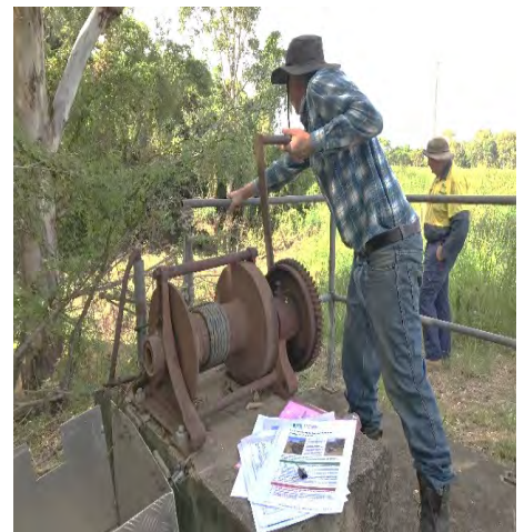
Landowner volunteer floodgate operator opening a floodgate
