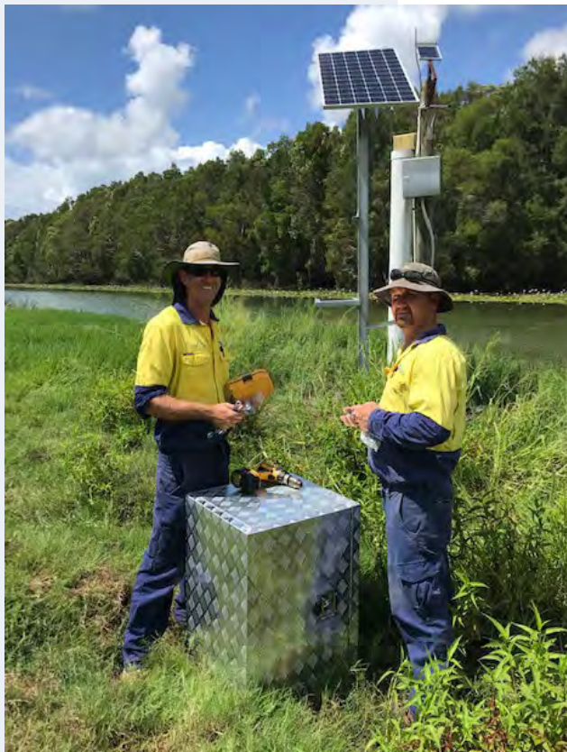
Rous Flood Mitigation Operators Installing a logger at the Tuckean
