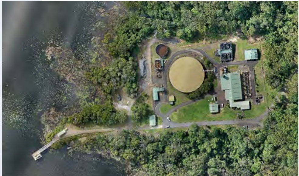
Nightcap Water Treatment Plant
