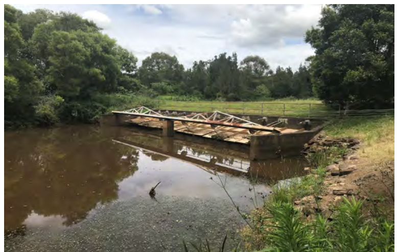
Rocky Mouth Creek floodgates
