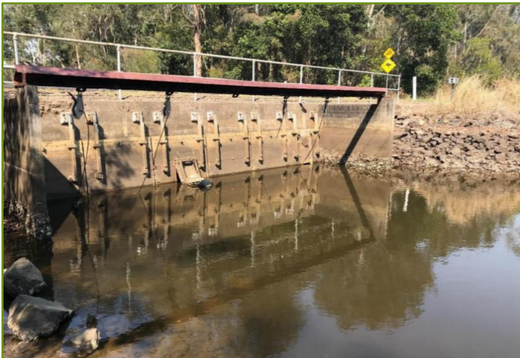
Keith Hall Floodgate
