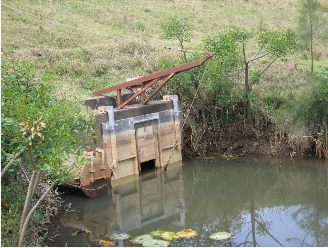
2: Wades Canal floodgates with sluice window open.
