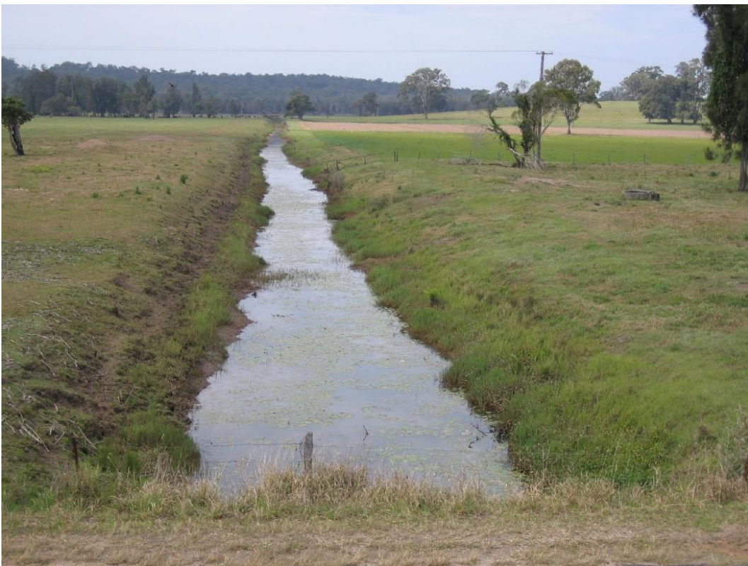
3: Wades Canal looking upstream from floodgates.
