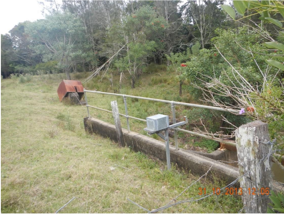
2: Sandy Creek No.2 floodgates, showing culvert headwall, lifting devices and handrail.
