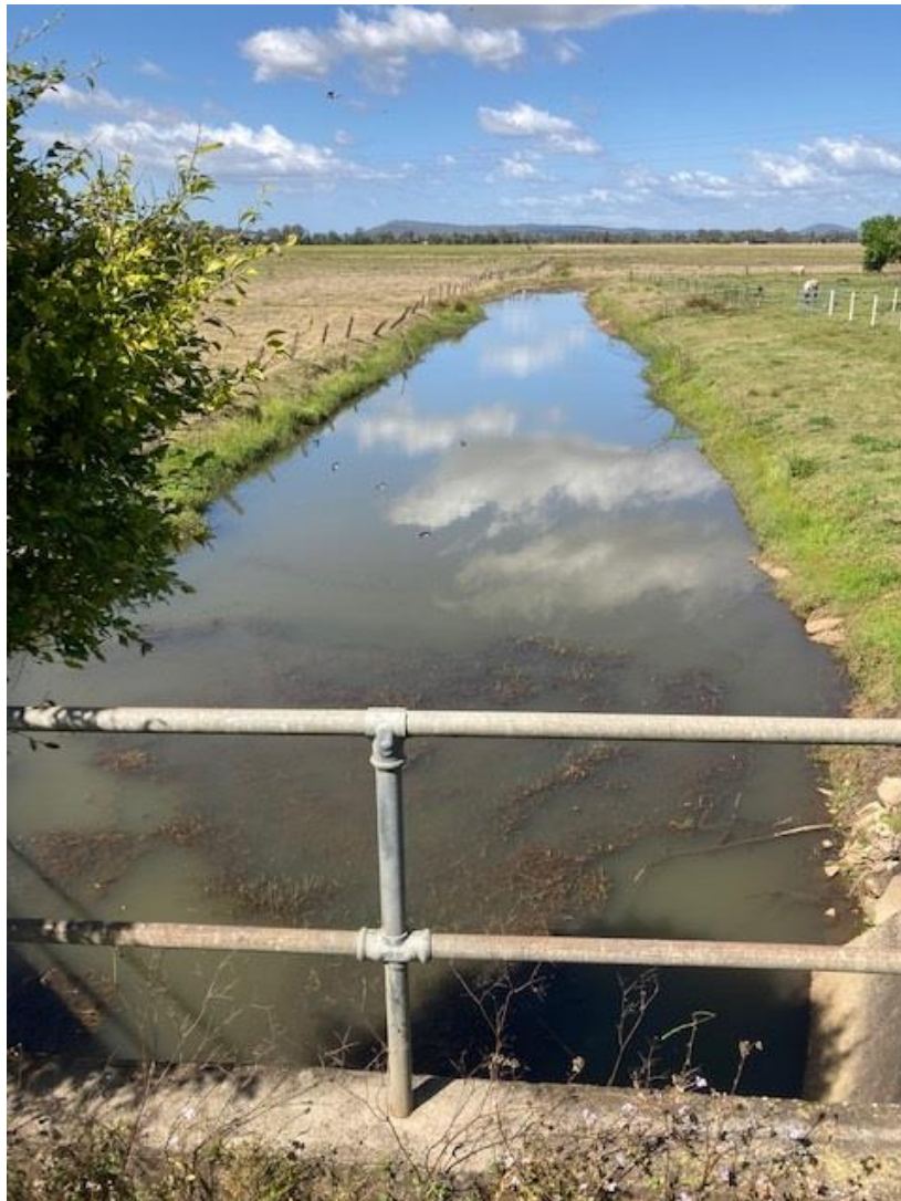
3: Looking up Sandy Creek No.2 drain from floodgates.
