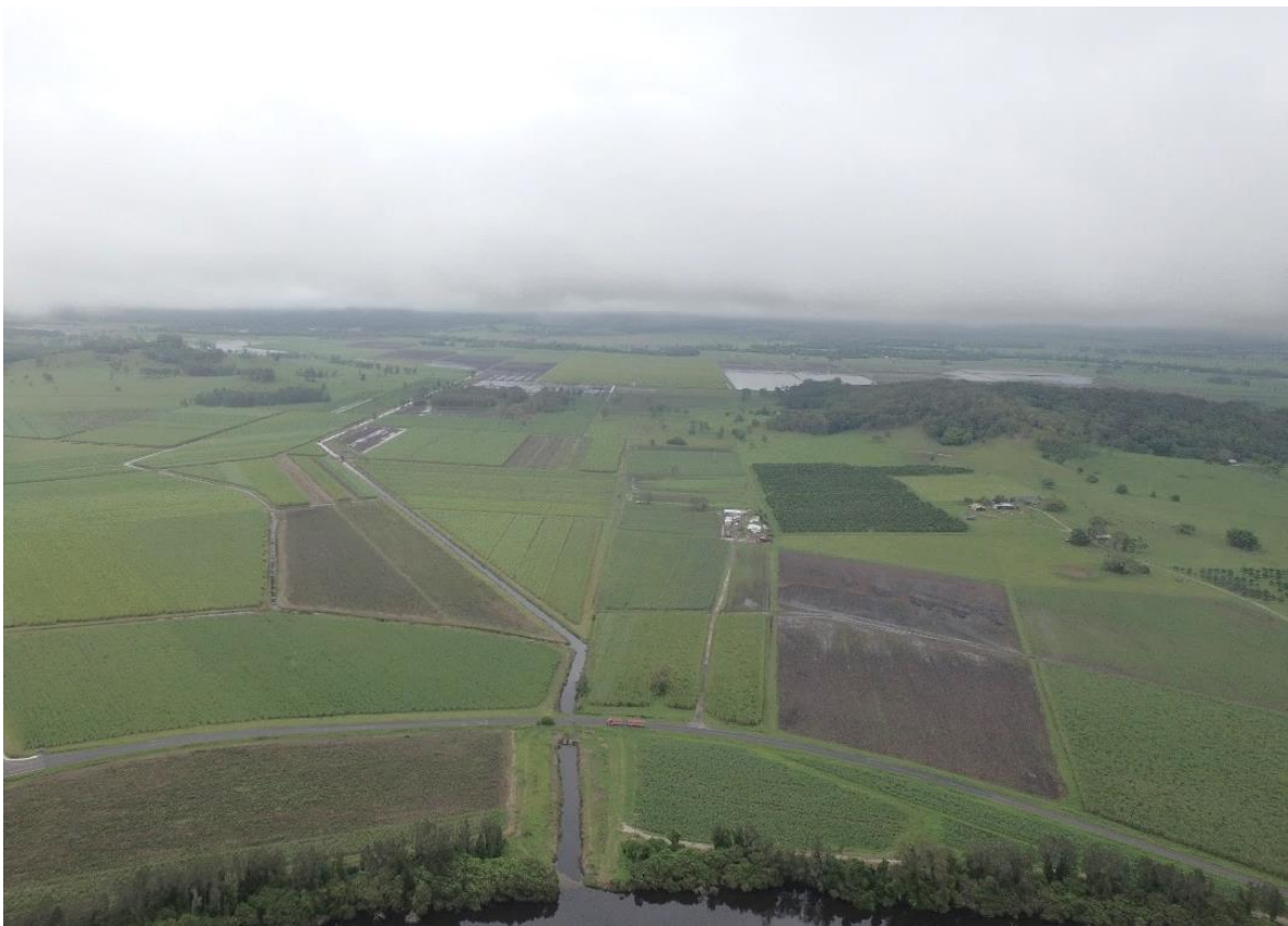
3: Aerial shot of Reardon's drain, looking upstream from floodgates after minor flooding in February 2020.
