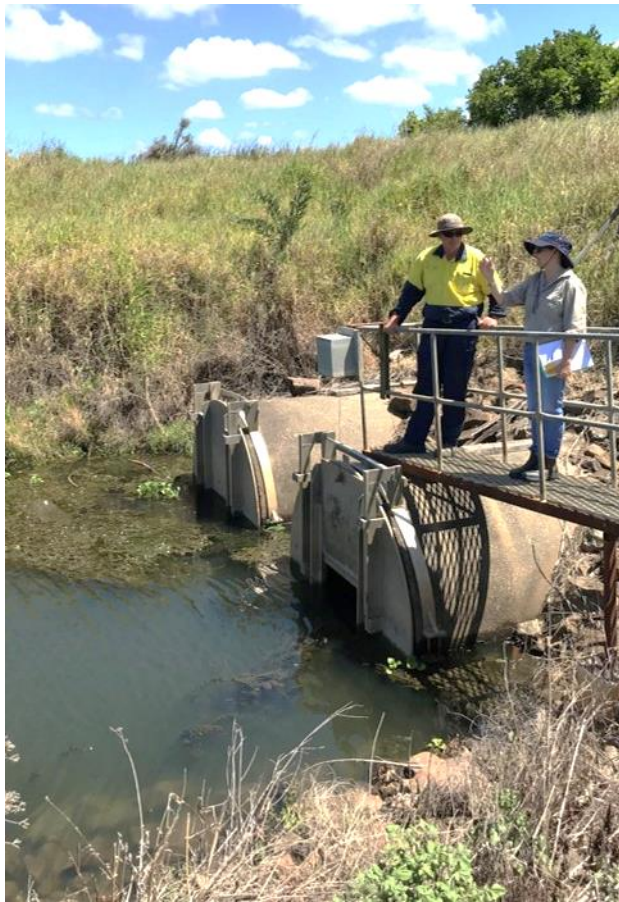
2: Reardon's drain floodgates, showing sluice window in a fully open position.
