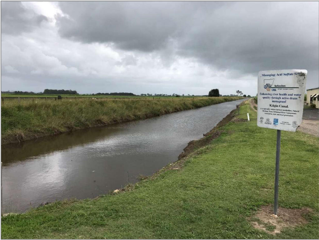
Figure 4: North Woodburn-Kilgin drain looking upstream from floodgates.
