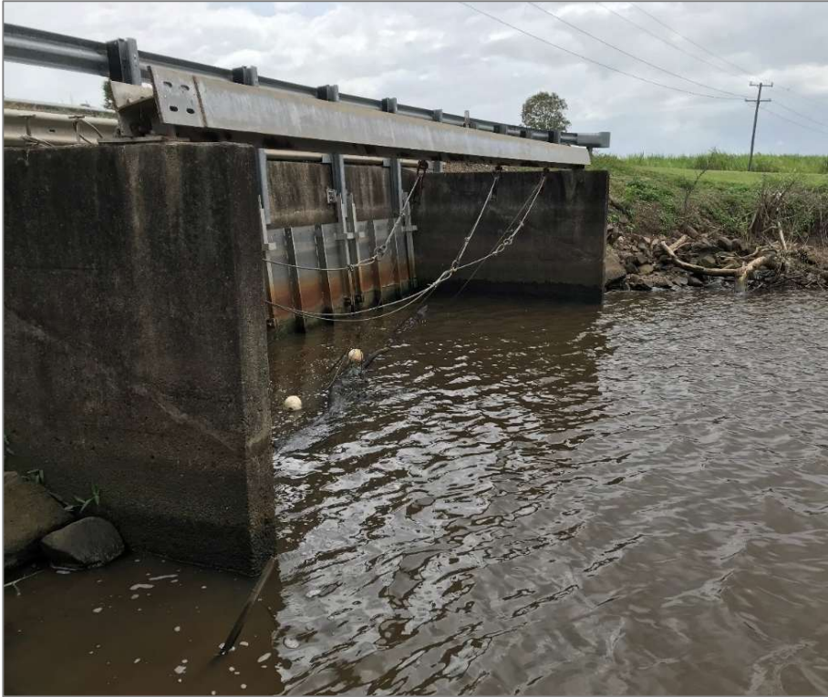
Figure 2: North Woodburn-Kilgin drain floodgates.
