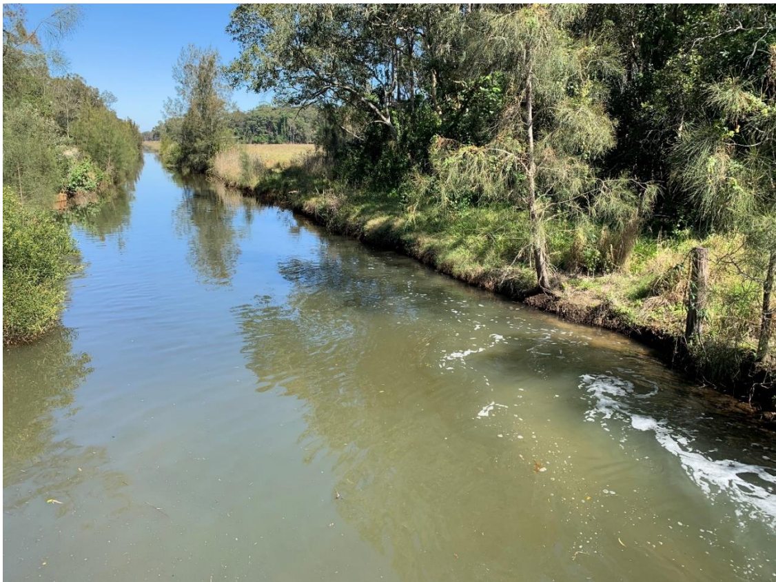
4: Keith Hall No.1 flood mitigation drain looking immediately upstream of the floodgates at Mobbs Bay. Note incoming tidal water through the sluice window.
