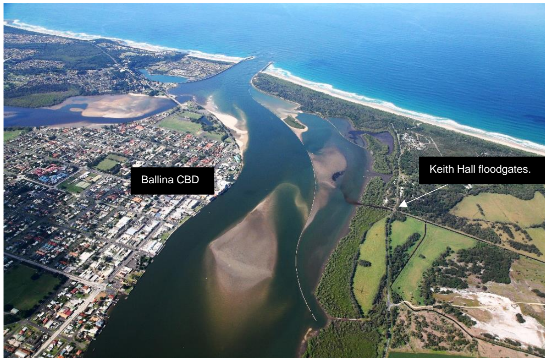
6: Aerial of KHDS discharging discoloured water into Mobbs Bay.
