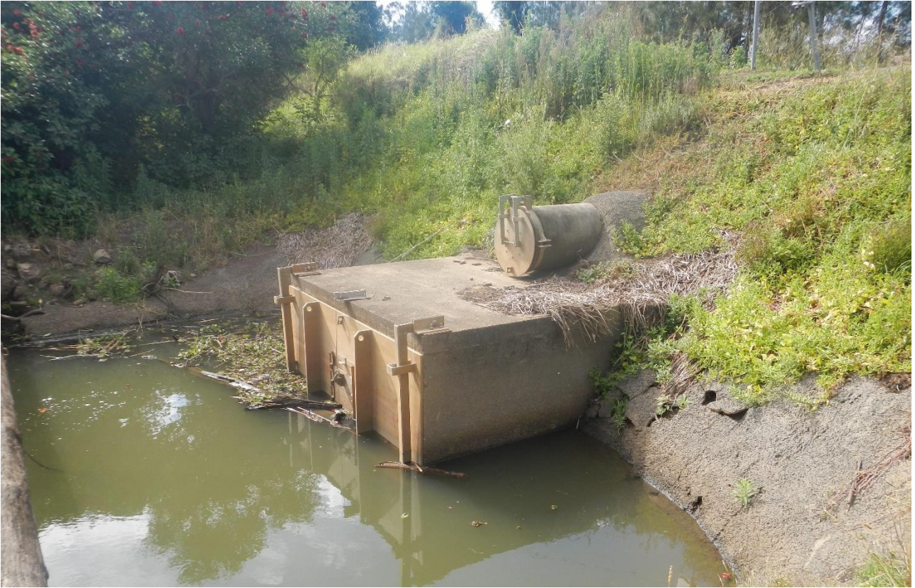
2: Campbell's Drain floodgates, showing sluice window.
