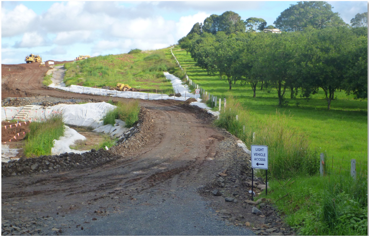
Figure 3-6 New Pacific Highway construction works, showing potential sediment sources.
