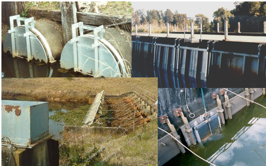
Clockwise from top left: Two round flap style floodgates - A 24m outlet with eight square flap style floodgates, three of which are fitted with sluice gates - Sluice gate fitted to square flap style floodgate - Six square flap style floodgates with lifting gear.
