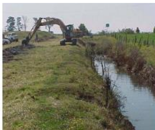
Sediment should be placed away from drain and positioned to avoid leachate running back into the drains and watercourse. (Source: Kempsey Shire Council).
