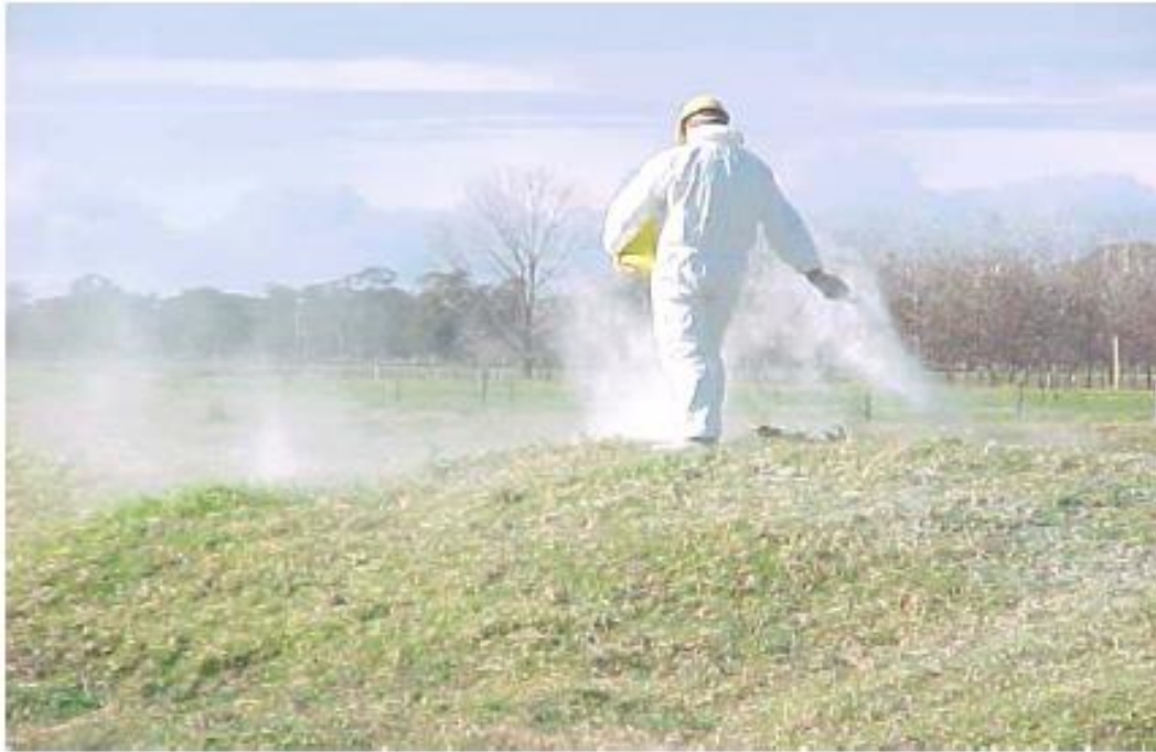
Lime being spread over area where spoil is to be placed. (Source: Kempsey Shire Council).
