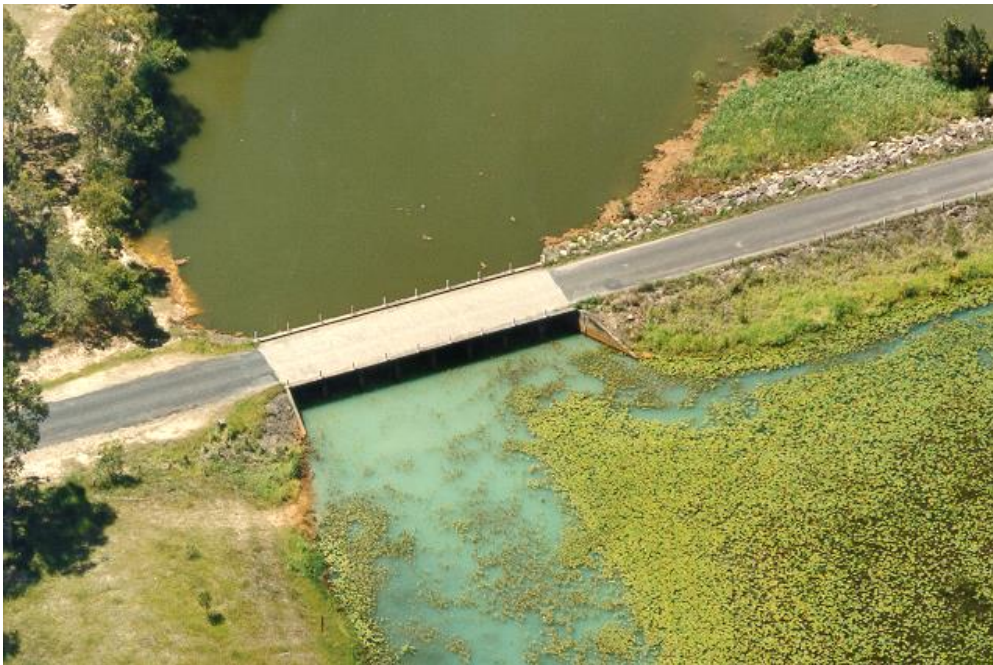
Aluminium flocculants in acid water behind the Bagotville Barrage, an indicator of acid sulfate soils. Photo taken prior to the implementation of tidal flushing.
