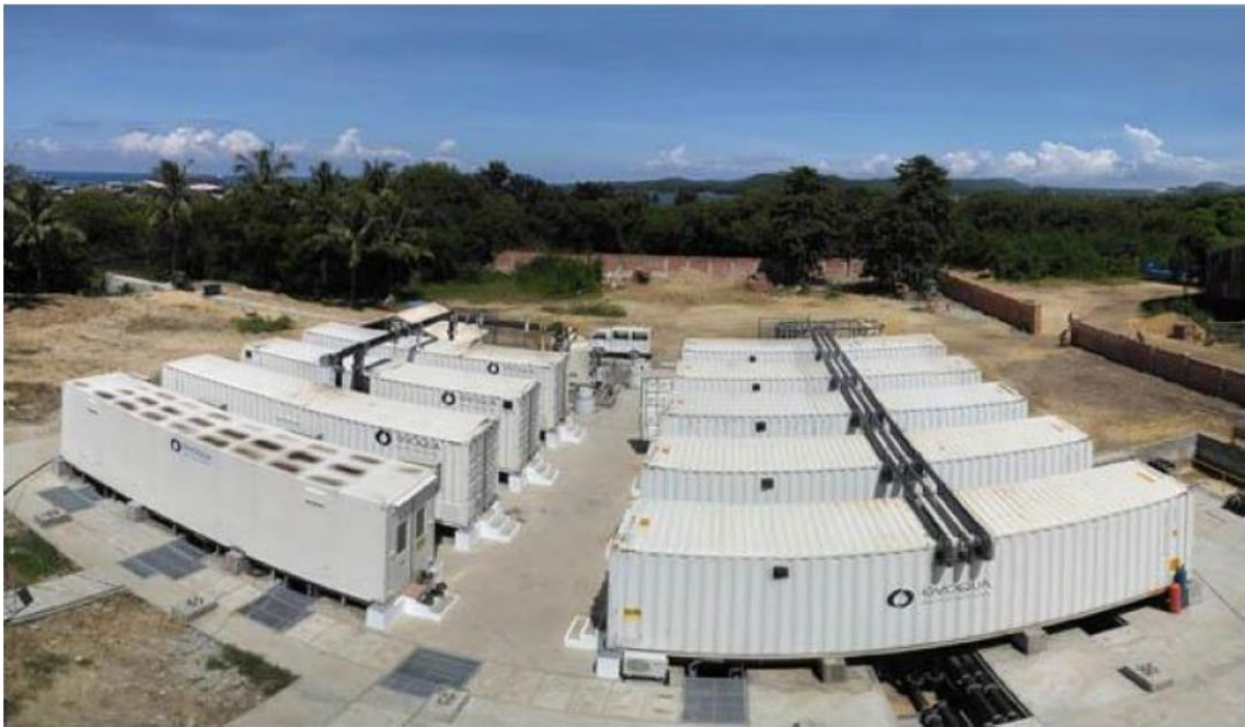
Figure 3-5: Semirara plant as built, 1,925 m 2 for 7 MLD (~418 m 2 /ML)
