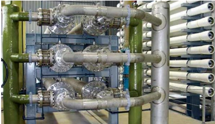
Figure 12. Photo of DWEER devices installed in desalination plant
