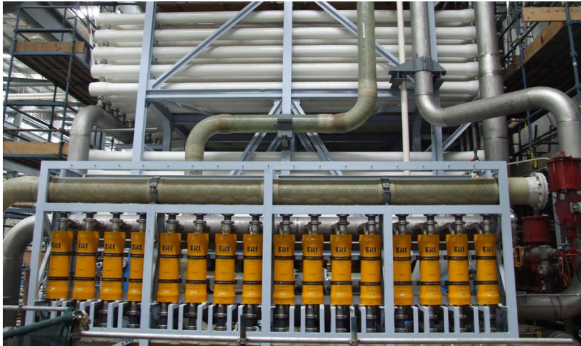
Figure 10. Energy Recovery Inc Pressure exchangers at Perth Desalination Plant
