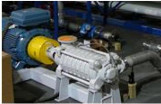
Figure 33 SWRO feed pumps
