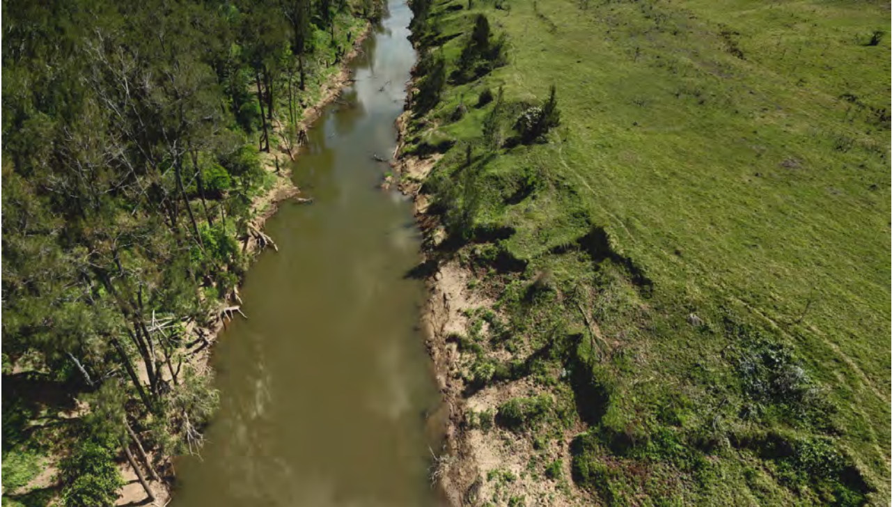
Figure 121. Example of the difference in bank erosion between a vegetated and unvegetated bank. Bank on right of image is showing evidence of toe scour coupled with mass-failure – rotational slumps. Bank on image left is primarily experiencing toe scour without mass failure
