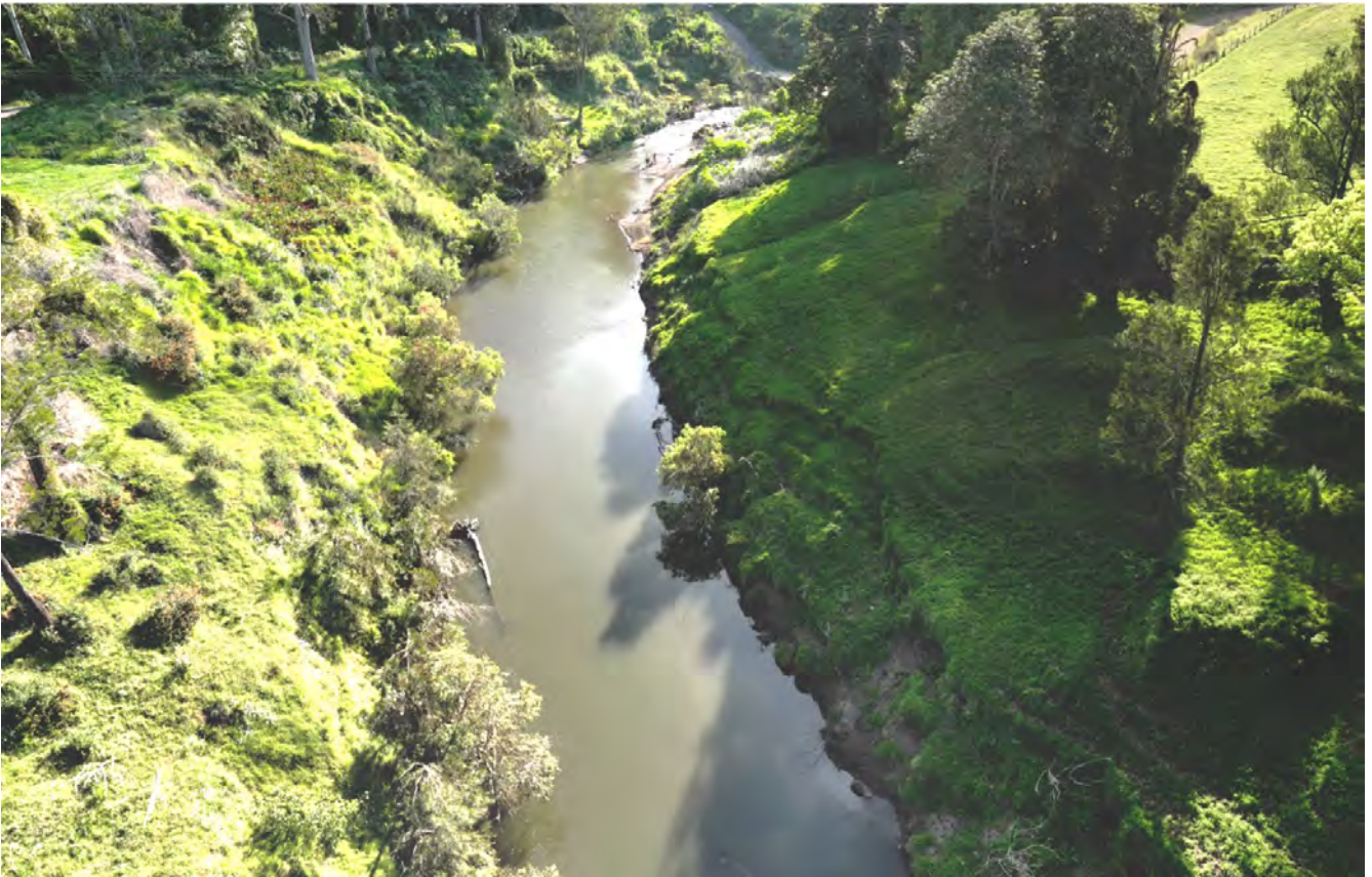
Figure 123. Example of a section of the upper Richmond R showing evidence for multiple rotational mass failures. Note the bank at right of image is showing evidence for toe scour – which has led to shallow mass failure – whereas the bank at left of image has good toe protection from a line of Melaleuca citrina. Note also it is clear that there are many old mass failure scars that have self healed.
