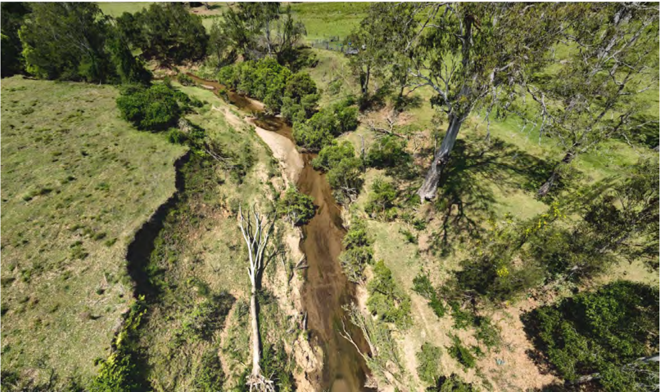
Figure 126. Further example of a section of channel that has experienced previous mass failure that is now partially restabilised by grasses and herbaceous vegetation. A site like this would respond extremely well to stock exclusion and assisted natural regeneration.
