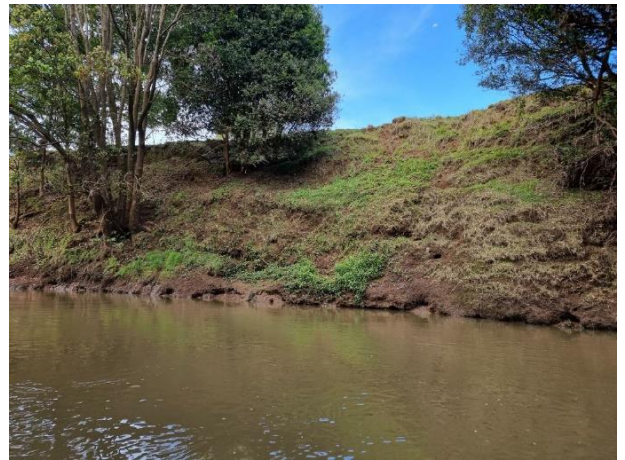
This picture shows bank toe cracking and slumping. This is evidence of incision.
