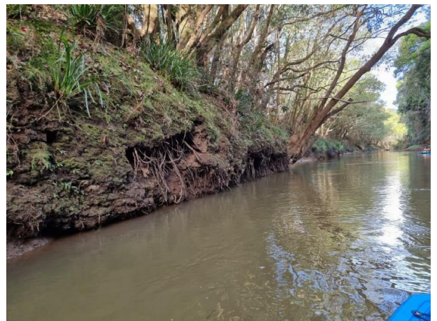
The channel is seen to widen here with toe scour exposing tree roots. Potential slumping.
