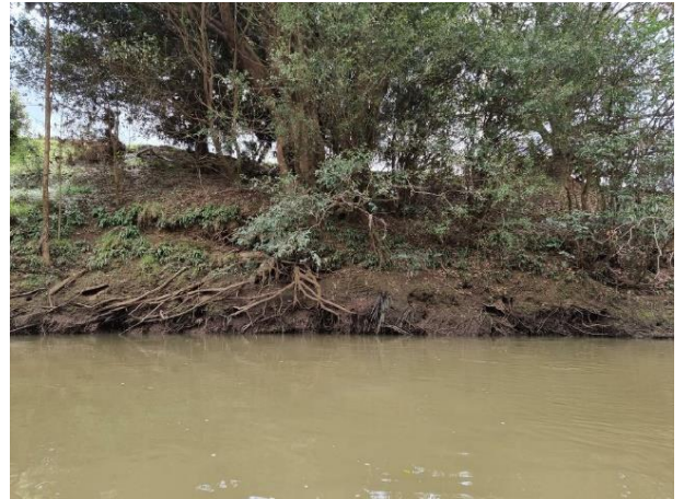
This photo shows toe and bank scour.
