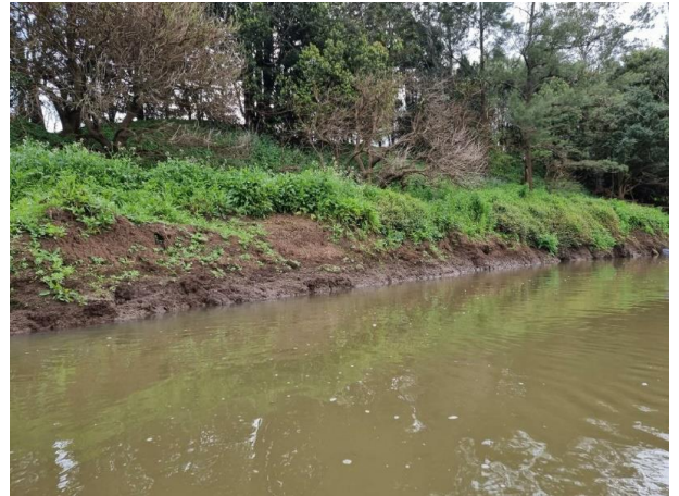
Toe failure and scour is seen here.
