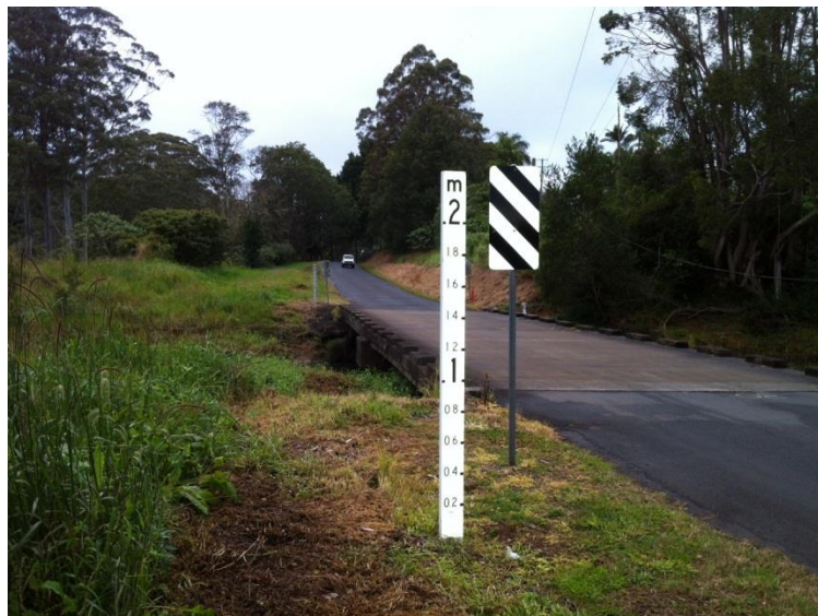
Figure 4-4 Flood depth road marker (Eltham Road)
